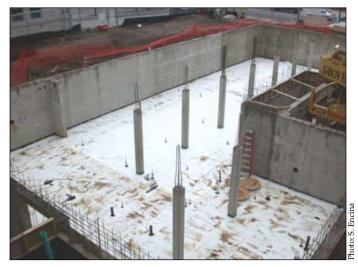
4. Finished basement with underslab waterproofing in place prior to having the basement floor poured.
