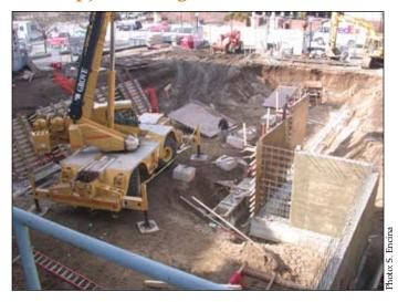
$2. \ Earth\ retention\ installation\ and\ forms\ being\ placed\ for\ basement\ concrete\\ wall\ pours.$
