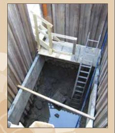
A view of the deep trench from above as the pump (slender blue tube just right of ladder) is working to drain the water.
