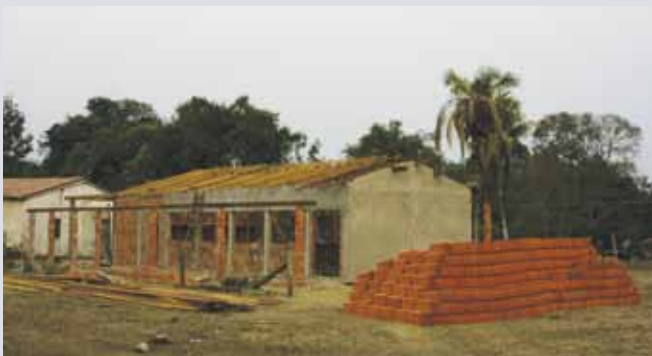
Pantanal School Building.
