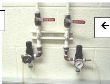
← Valve for nitrogen cavity purge
