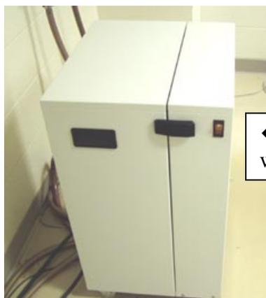
← On / Off switch for water chiller
