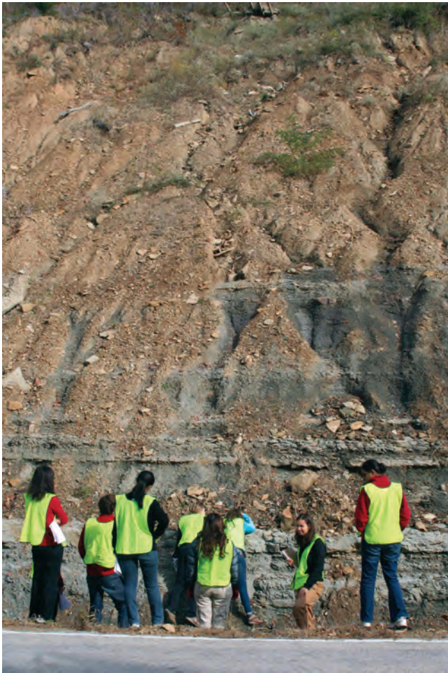
Above: Landslide Destruction. Students calculate failure probabilities of a shallow landslide in Northeastern Kentucky that was activated after road construction changed the hill-slope angle; the landslide damaged or destroyed several homes in the spring of 2010.
